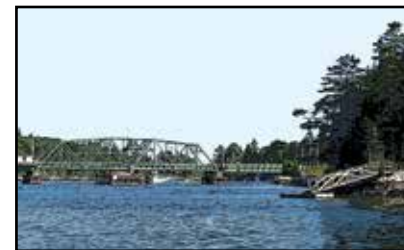
Swing bridge connecting Southport & Boothbay Harbor
